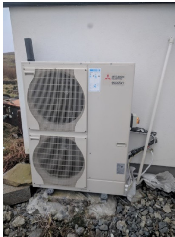
Mitsubishi Electric air to water heat pump
