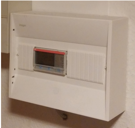
Electricity meter, 3 phase, ABB B23 113-100
