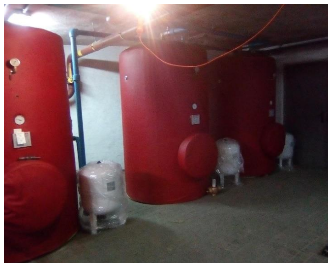
Figure 41: New thermosolar system water tanks
