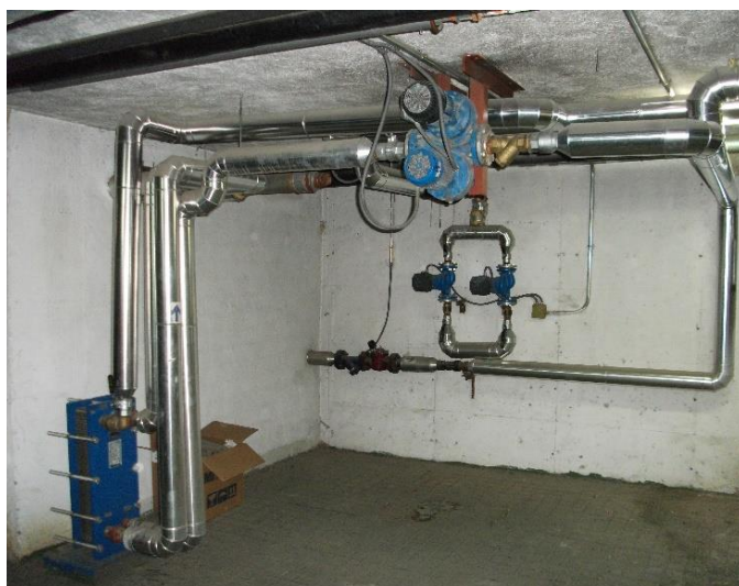
Figure 42: Original DHW pipelines
