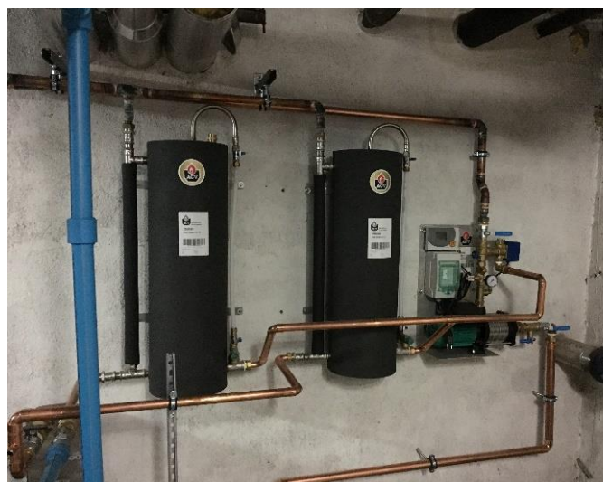
Figure 43: New thermosolar system pipelines
