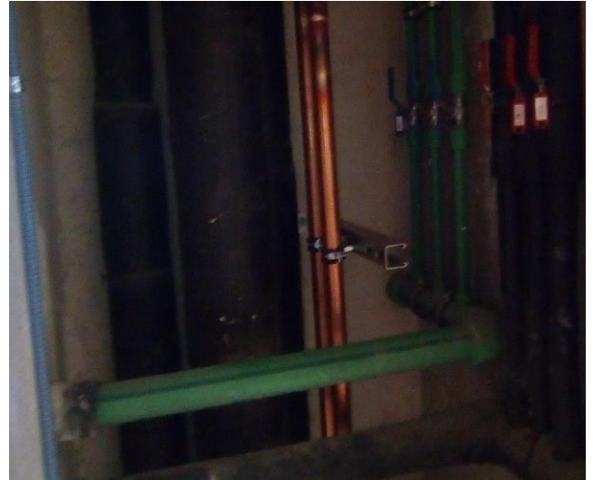
Figure 34: Thermosolar system pipelines
