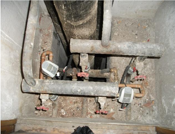
Figure 33: Vertical hole for thermosolar system pipelines
