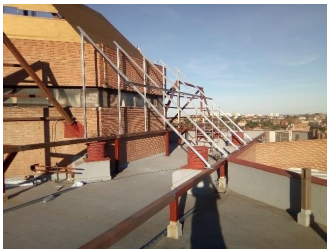
Figure 32: Additional new structure for solar collectors
