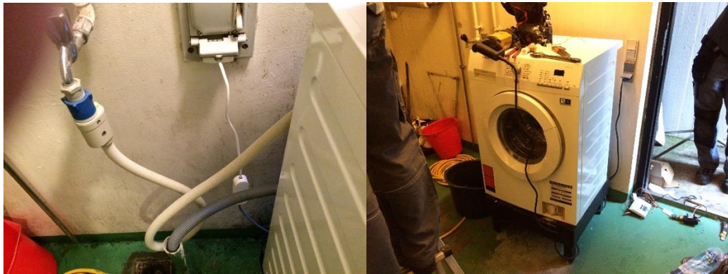
Figure 16 Develco Smart Cable – Washing Machine
