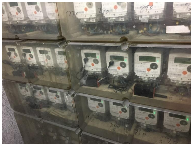
Figure 28: Ene's optosense devices deployed in company meters
