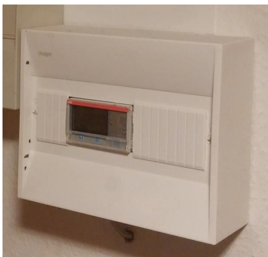
Electricity meter, 3 phase, ABB B23 113-100
