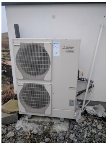
Mitsubishi Electric air to water heat pump
